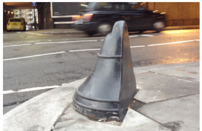
CAST IRON TRAFFIC BOLLARD WEIGHT: 120KG
